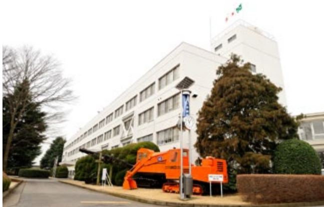
Tsuchiura Works East Building and the Hitachi UH03 hydraulic excavator, which is included in the list of Japan's Mechanical Engineering Heritage.
